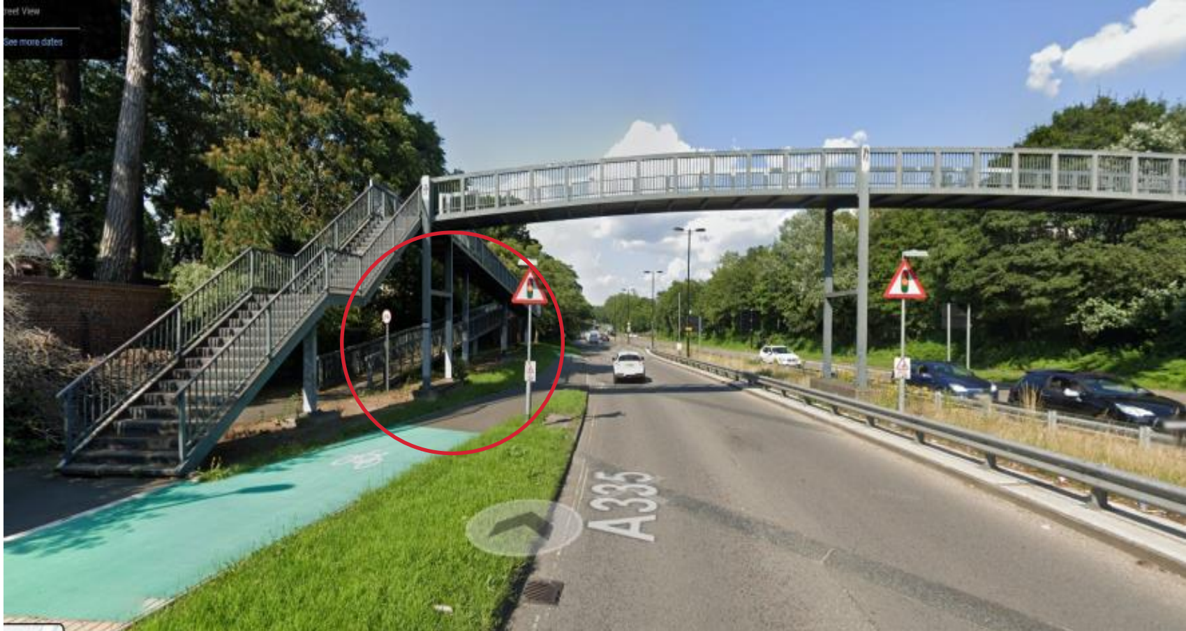
Pedestrian footbridge with ramps in Southampton, UK (Source: Googlemap, 2023)
