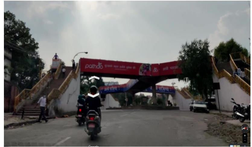
Pedestrian footbridge at Ratnapark, Kathmandu (Source: Googlemap, 2023)
