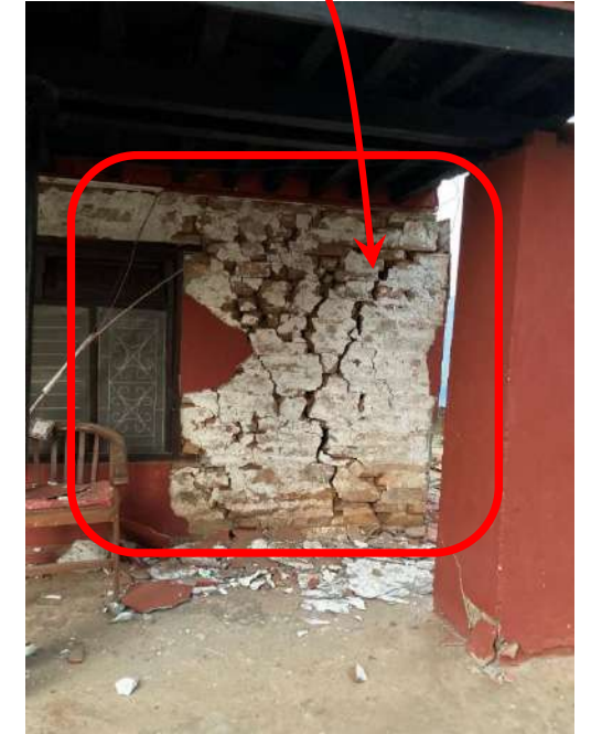
Wall pier diagonal cracking
