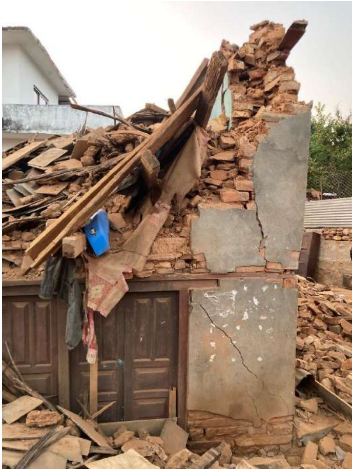
Complete collapse of Stone Masonry Building in Mud Mortar at Khalanga, Jajarkot
