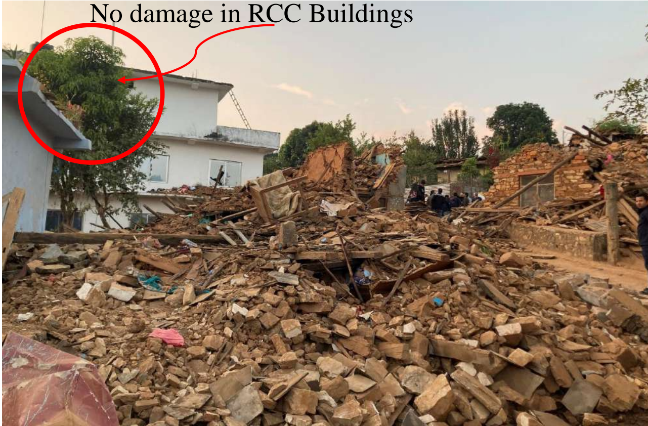
Collapse of Stone Masonry Building in Mud Mortar at Khalanga, Jajarkot
