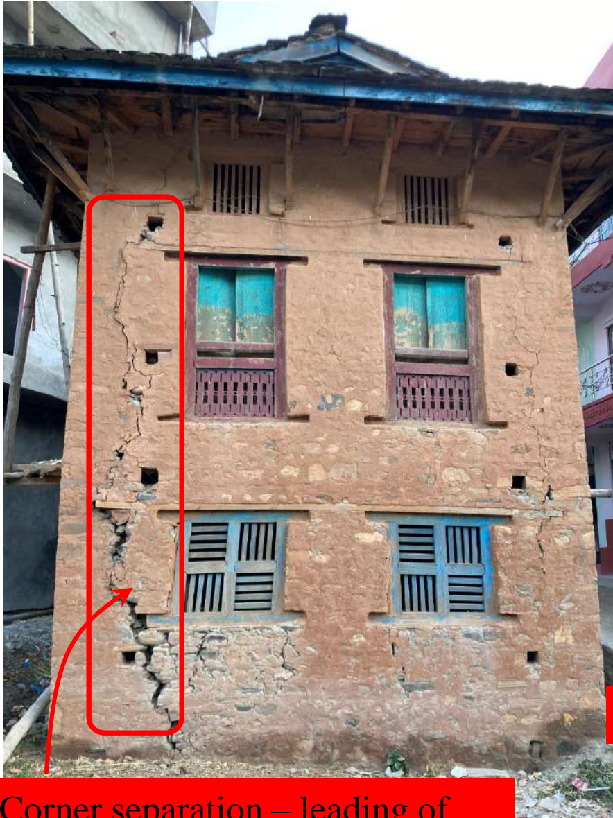
Vertical cracks at corners
