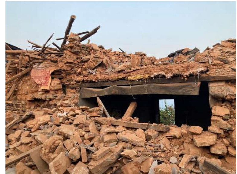
Complete collapse of Stone Masonry Building in Mud Mortar at Khalanga, Jajarkot
